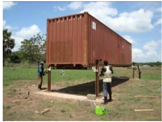
Container being lowered on “lifting jacks”
