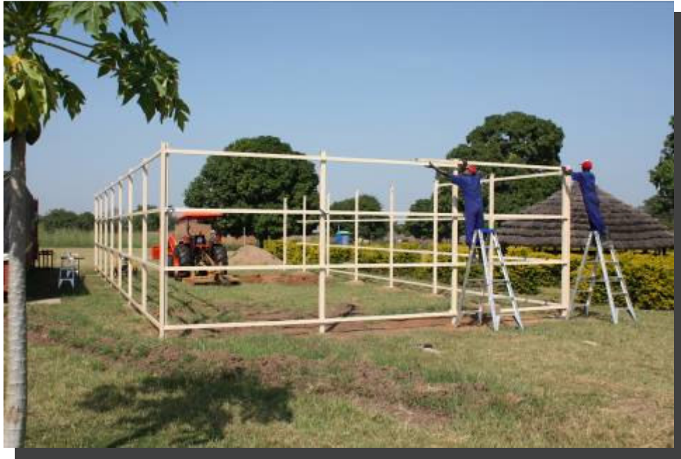
Workshop under construction: November 24 th 2011
