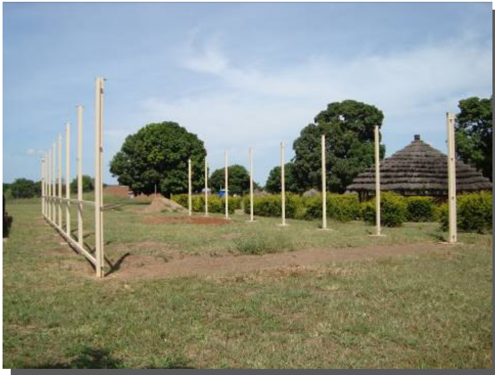
Workshop under construction October 2011
